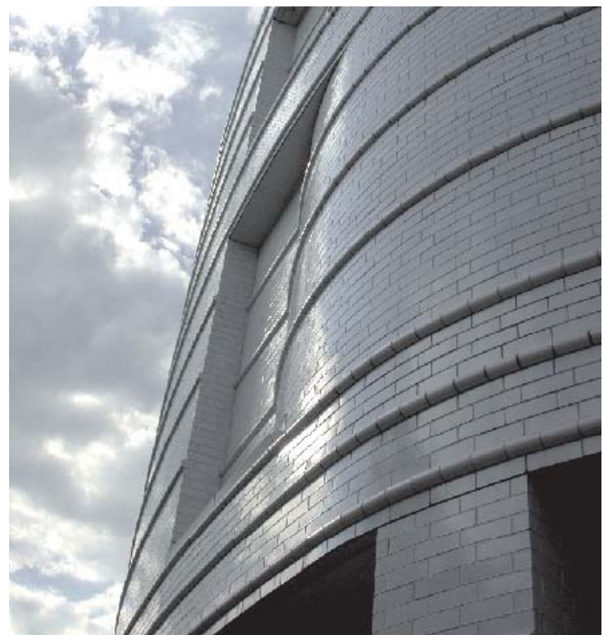
Photo 1 Glazed Brick Used for Entire Facade
