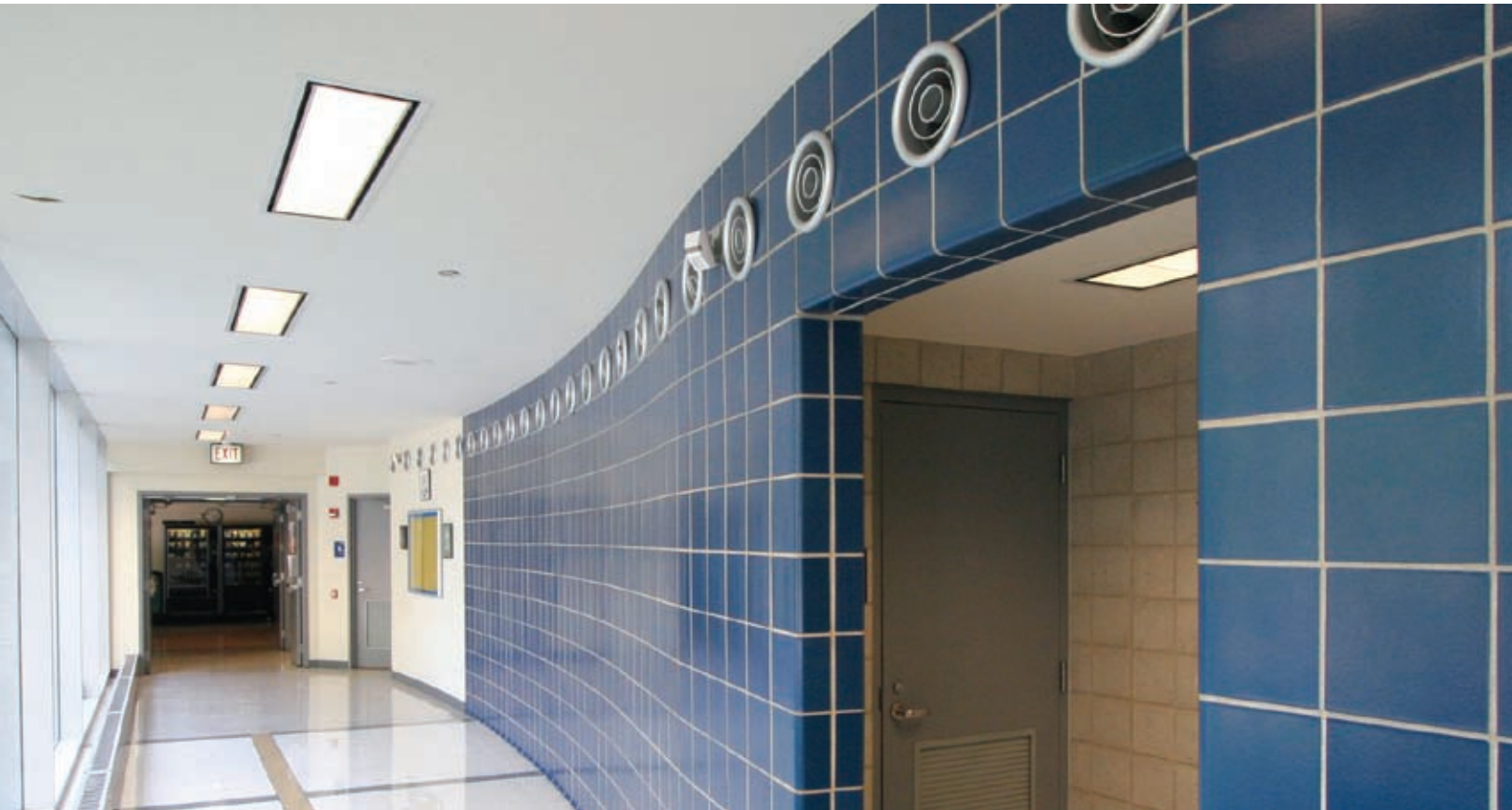
Structural Glazed Tile; Little Village High School – Chicago, IL
